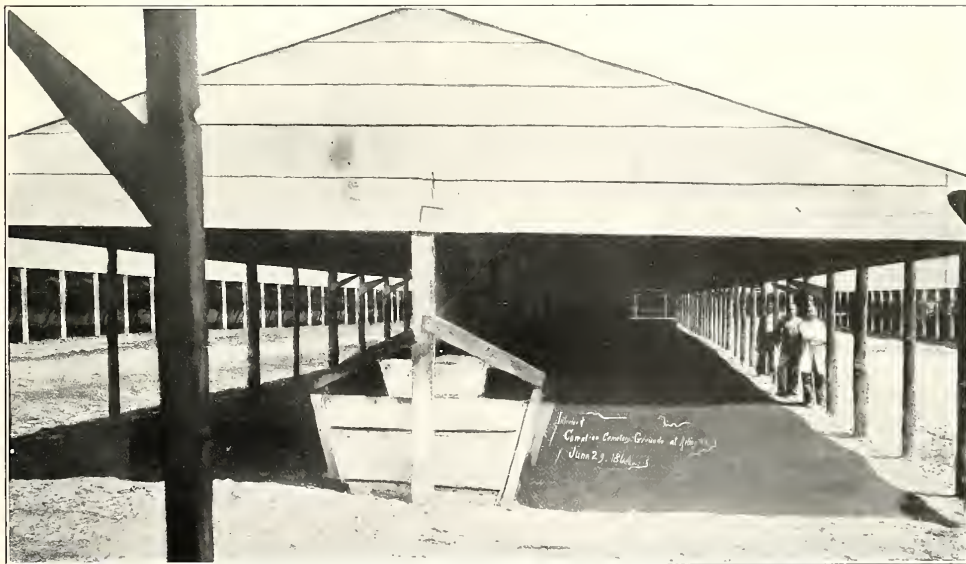
INTERIOR VIEW OF CAVALRY STABLES AT ARLINGTON
